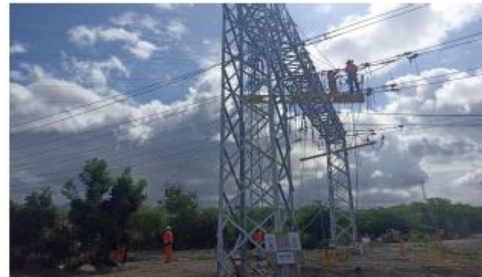
MV LINE CABLE PULLING
