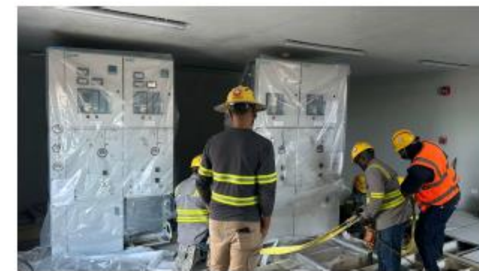
SWITCHING CENTER EQUIPMENT INSTALLATION
