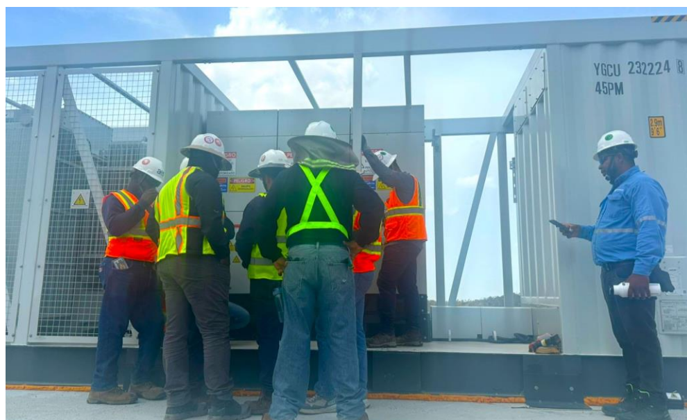
O&M TEAM INVERTER PRACTICAL TRAINING
